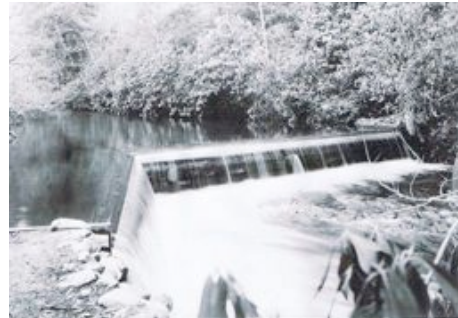
Figure 5. Forge Creek Dam After 1930s Restoration
