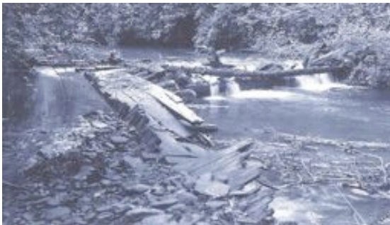
Figure 4. Forge Creek Dam Prior to 1930s Restoration
